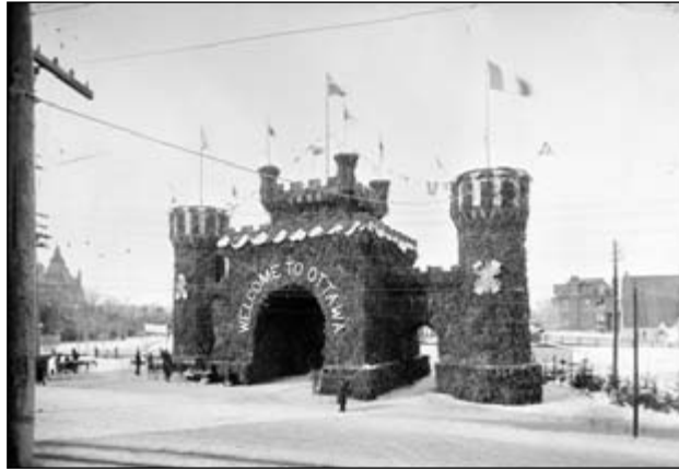
FIGURE 4: Mackenzie Avenue Arch. Courtesy of Library and Archives Canada [MIKAN 3401331].
