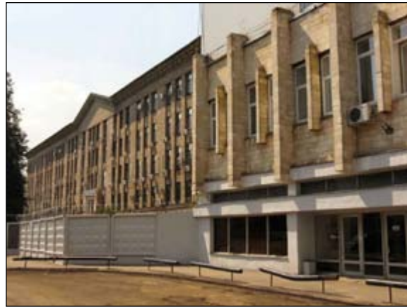
ADAMAS facility where the Olympic medals were manufactured
